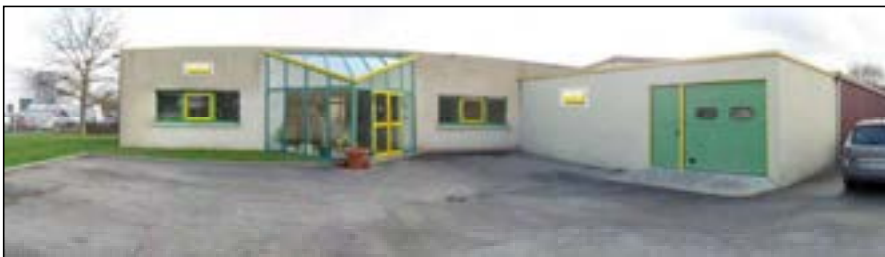
A.M.I. Building at Saint-Marcel (France)
